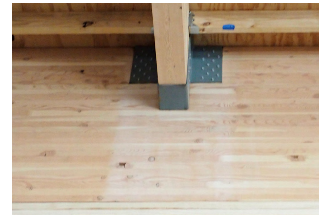
Figure 74 An example of color differences in the wood observed after staining was removed via sanding.
