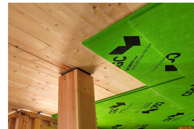
Figure 6 Fire-rated gypsum installed on the underside of the CLT floor mid-construction.
