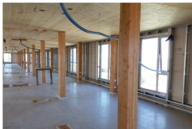
Figure 62 A temporary roof drain connected to hosing that directs the water outside.
