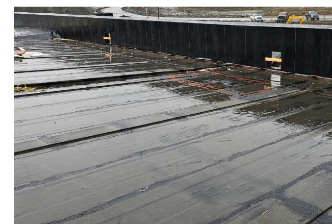
f) Vapor-impermeable self-adhered SBS roofing base sheet.
