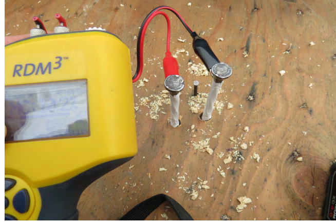
Figure 67 Moisture content reading taken through the panel spline using a moisture meter with extension pin probes.
