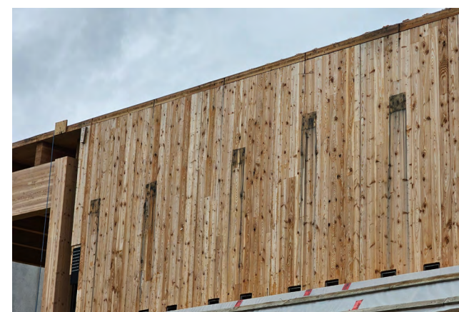
Figure 24 Water staining on mass timber wall due to excessive rainwater runoff from the roof wetting the face of the wall panel.
