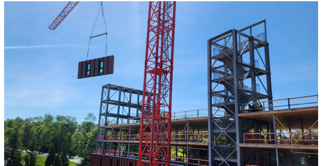
Figure 43 Prefabricated facade walls being hoisted into position for installation.
