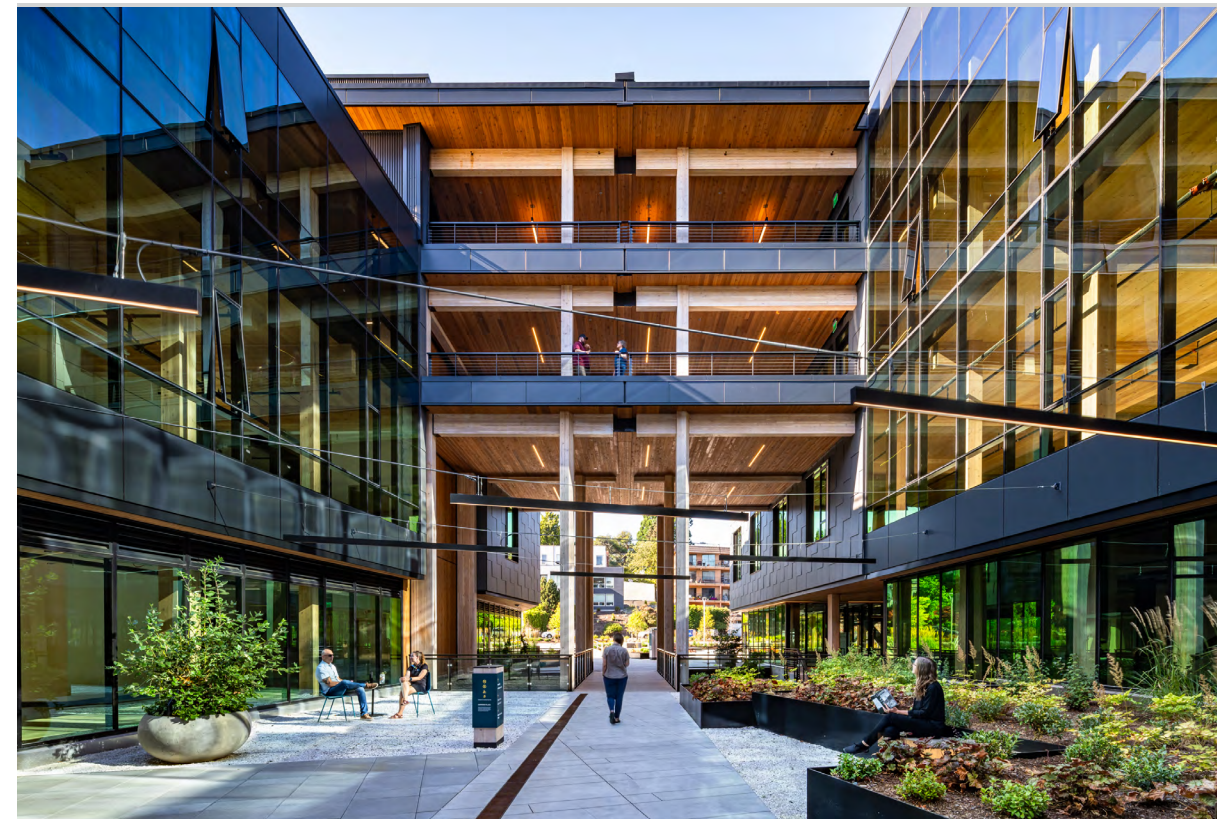
Figure 80 The open and exposed bridges showcase the beauty of the CLT and glulam. Image by Built Work Photography.
