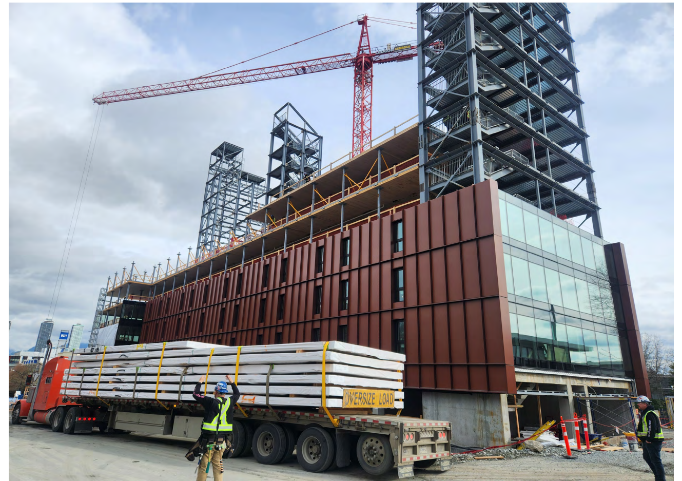
Figure 77 CLT floor panels delivered on-site for installation of the next level.
