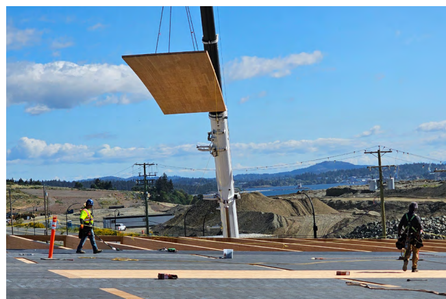
Figure 46 CLT panel with factory-applied protection being craned into position.
