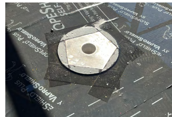
Figure 78 Drain port stripped in with tape/self-adhered membrane.
