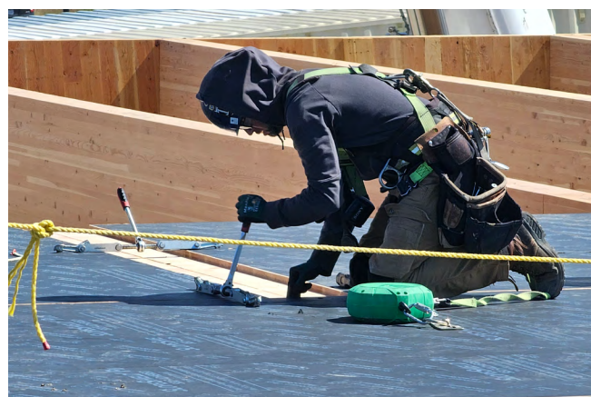
Figure 47 A mass timber installer securing the CLT panel placement.
