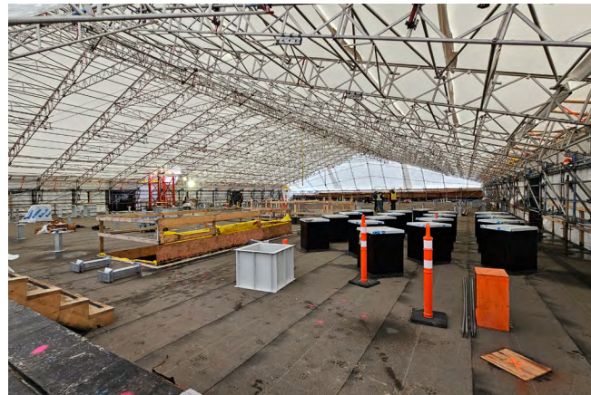
Figure 55 A tent installed over the roof of a mass timber building.
