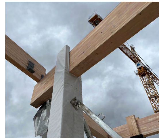
Figure 81 Glulam beams during construction.
