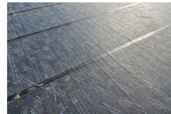
d) Vapor-permeable self-adhered membrane.
