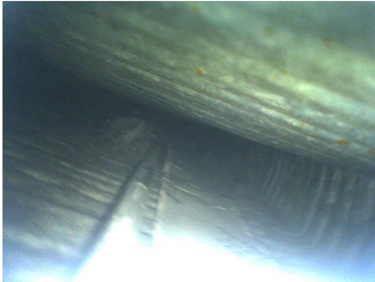
Figure A.1: Photo of the dryer exhaust duct at site A taken during sensor installation.
