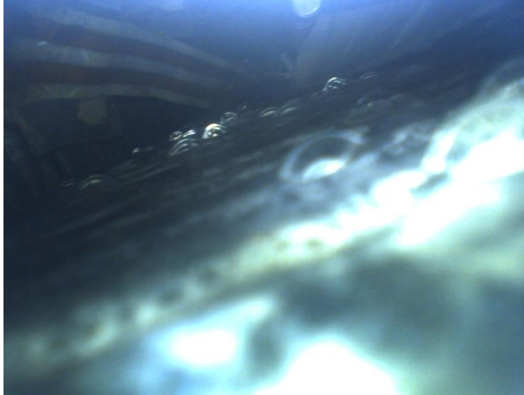
Figure A.10: Photo of moisture build-up at Site C, observed during sensor takedown.
