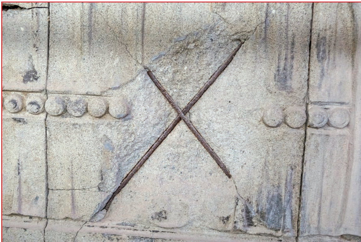
Figure 4 – Damaged cast stone due to corrosion of embedded reinforcing steel.
