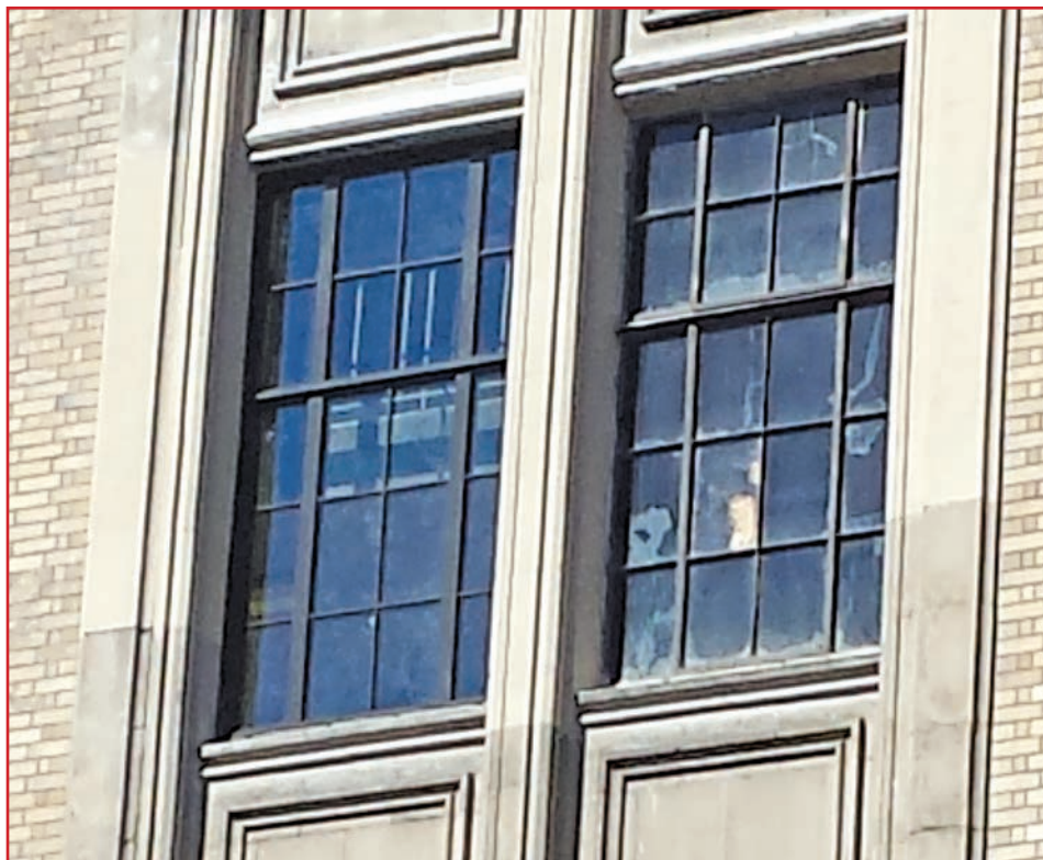
Figure 5 – Photograph of a new window on the left and an original window on the right.
