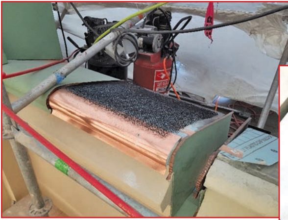
Figure 9A – Pre-patinated copper flashing installation on parapet walls. The wind clip is formed from new copper, and drain mat is installed below the cap flashing to facilitate drainage.
