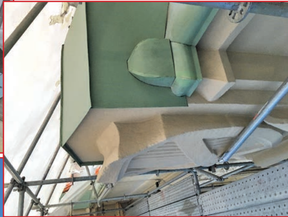
Figure 9B – Pre-patinated copper flashing installation on parapet walls.
