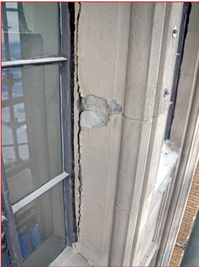
Figure 3 – Damaged cast stone due to corrosion of window frame and significant vertical compressive loads created by corrosion of the shelf angles at the floor levels.
