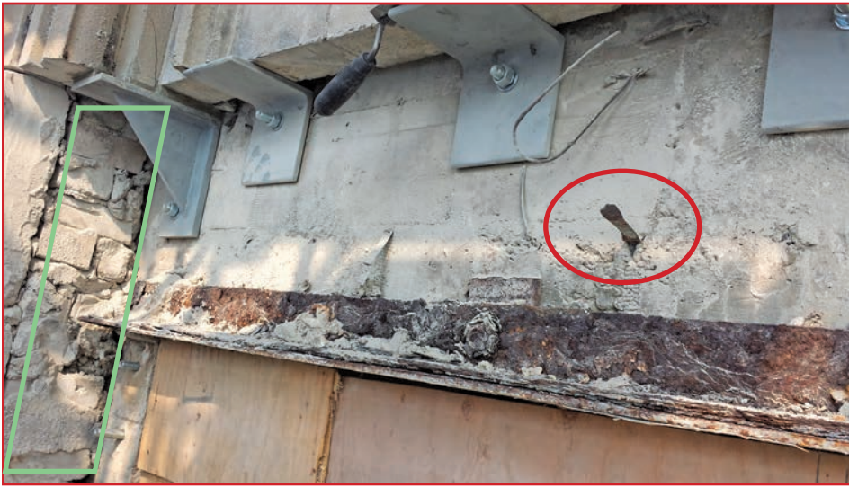
Figure 2 – Severely deteriorated shelf angle. The red circle illustrates one of the original masonry ties used to secure the cast stone to the concrete frame. The green rectangle illustrates the typical masonry rubble installed between the cast stone and the concrete frame. The plywood was used to protect the window during removal of the masonry.
