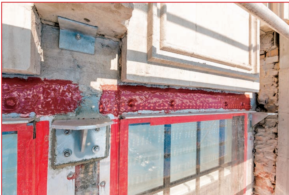
Figure 8 – Shelf angles attached to primary frame with anchors set into epoxy resin. Liquid-applied membrane used between shelf angle and concrete back frame.
