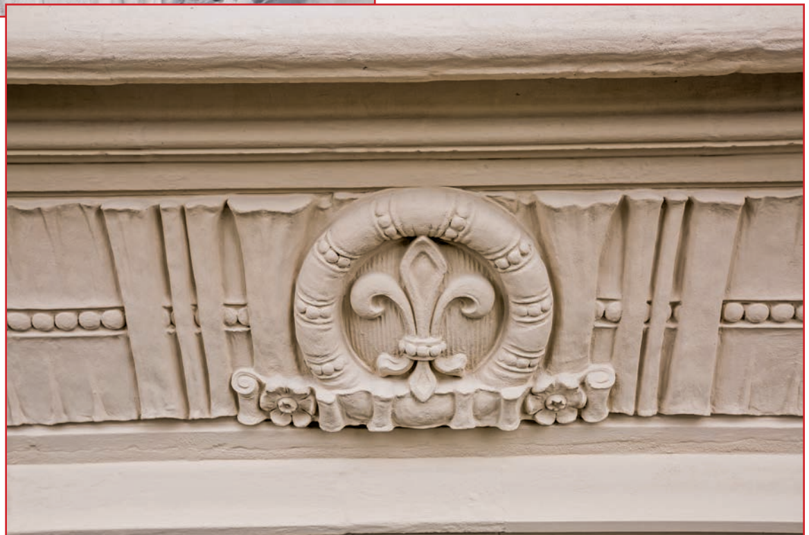
Figure 6B – Condition of cast stone after restoration.
