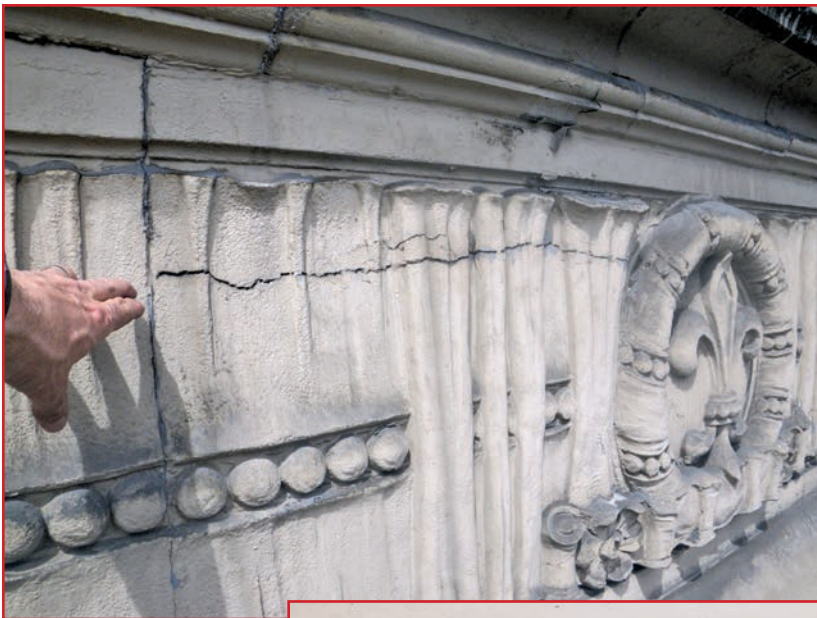
Figure 6A – Condition of cast stone at time of condition assessment.
