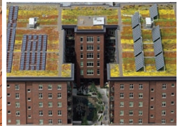
ABOVE At 31,597 ft 2 , this was the largest contiguous ecoroof in Portland in 2011. The roof is planted with drought-tolerant native species, has PV panels on the south half and solar water heaters on the north half.
