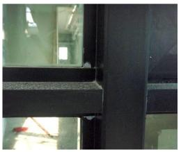
Figure 1: Typical chipped paint on a vertical mullion at the intersection with the horizontal mullion.
