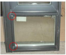
Figure 2: Example of chipped paint on the left frame member but not the right.
