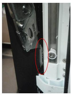
Figure 7: Inside of the jamb extrusion on an operable vent frame. This paint flaked off with a fingernail.
