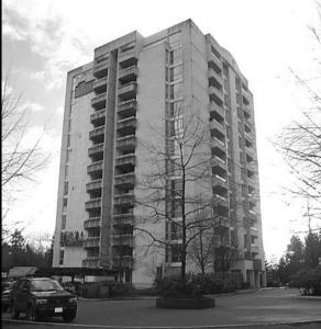
Photo A-1: Stucco cladding fell from north side of this high-rise building during high winds in late November 1998. The yellow indicates new sheathing in the area where cladding fell.
