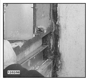
Photo A-2: Wet gypsum board sheathing, corrosion of steel studs and fasteners result in lower capacity of attachment. When combined with high winds (considerably below design loads) failure occurred.
