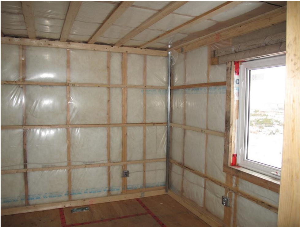
Figure 2 – Photograph of a 2x6 wood frame wall in Yellowknife with batt insulation and polyethylene and interior 2x2 cross strapping for interior insulation (Photo: Larry Jones)
